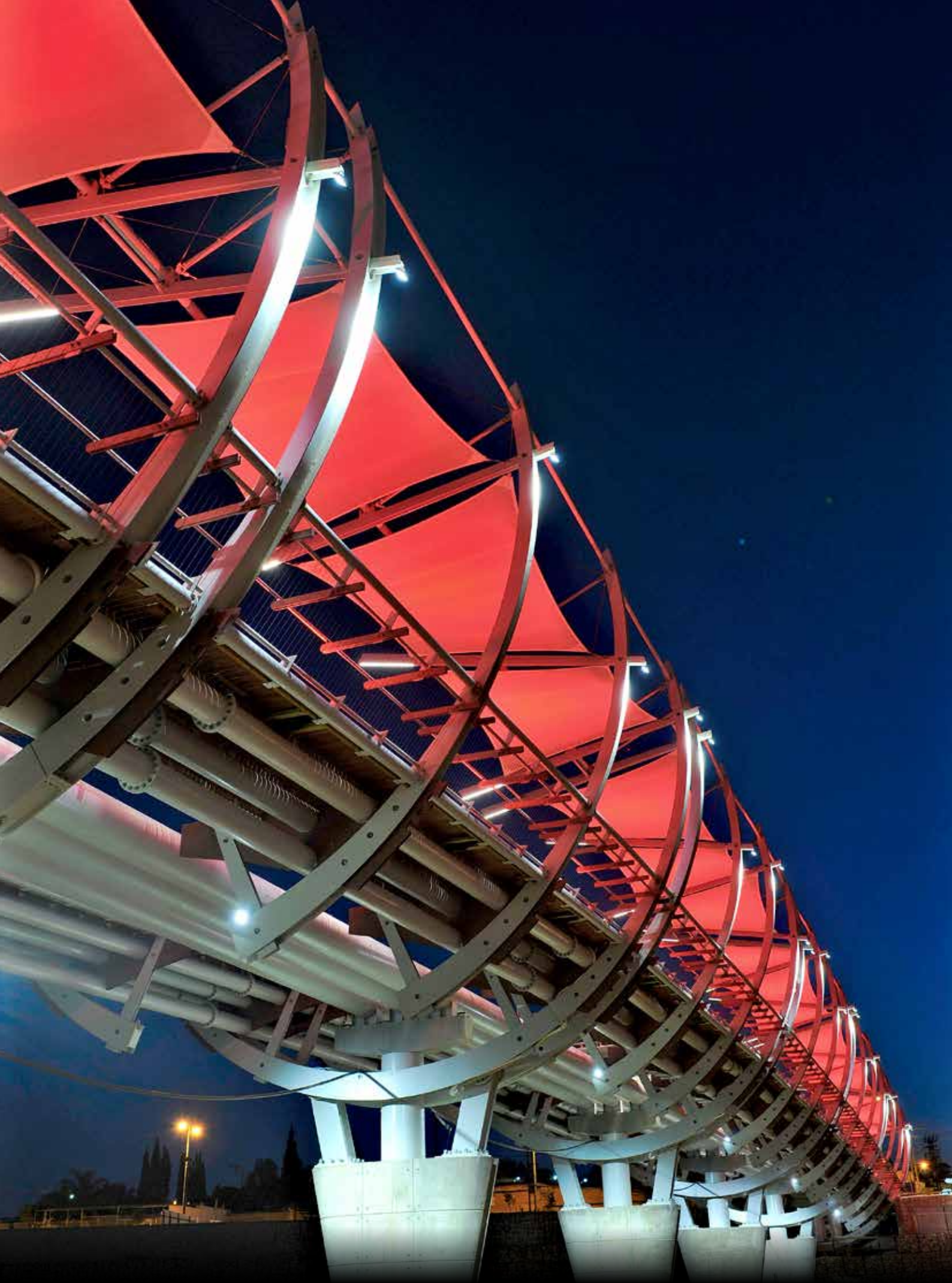
Pipe Bridge - Be'er Sheva, Israel
